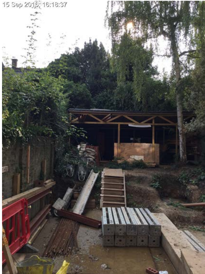
View from 97 Randolph Avenue towards the proposed location of mechanical plant.
